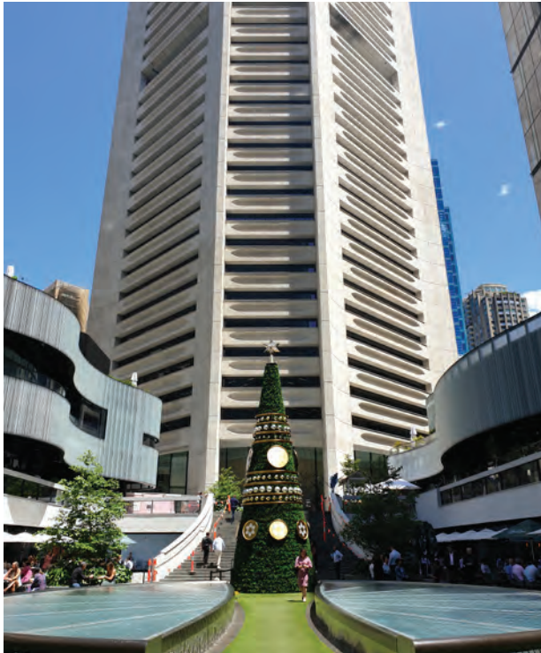
ACICA's new office space is located in 25 Martin Place
